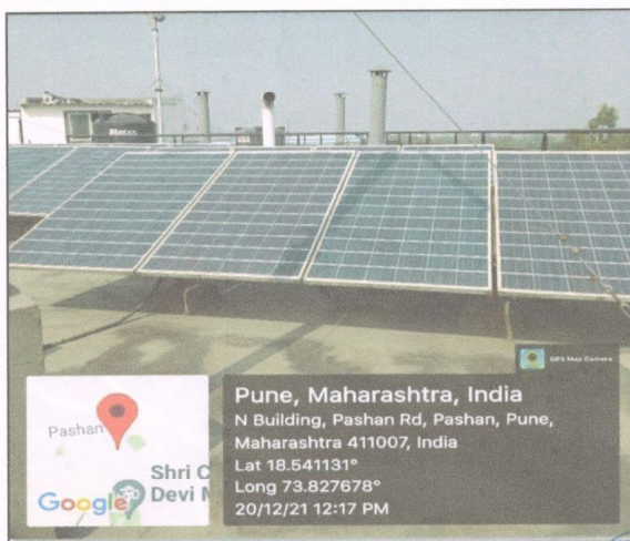
Photograph of 15 kWp Roof Top Solar PV Plant:
